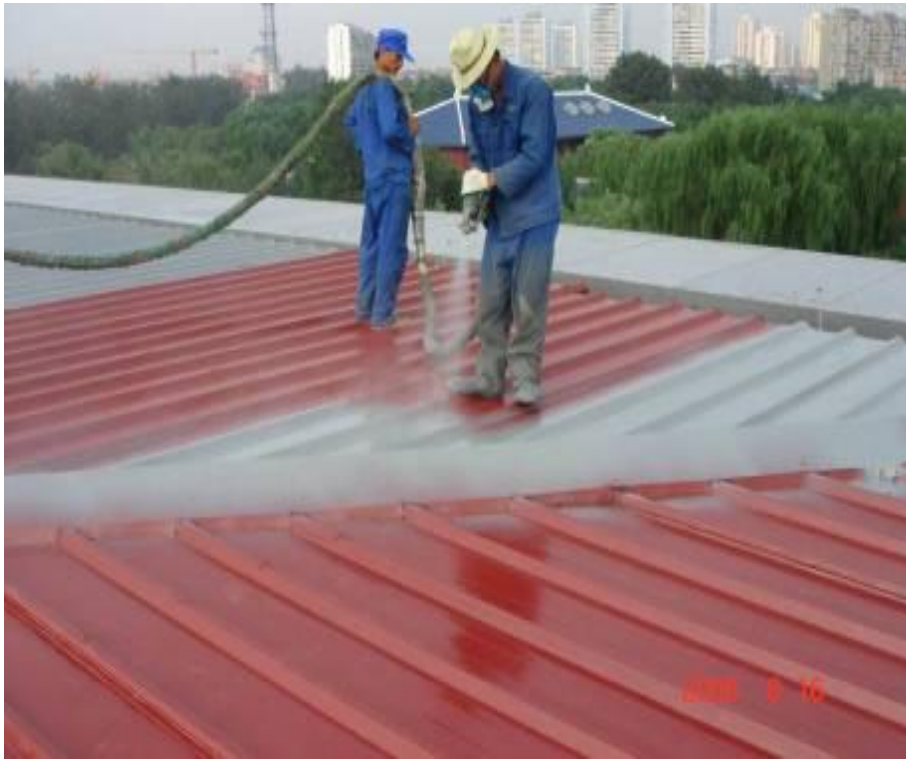
Beijing Wanfangting park Roof water-proofing
