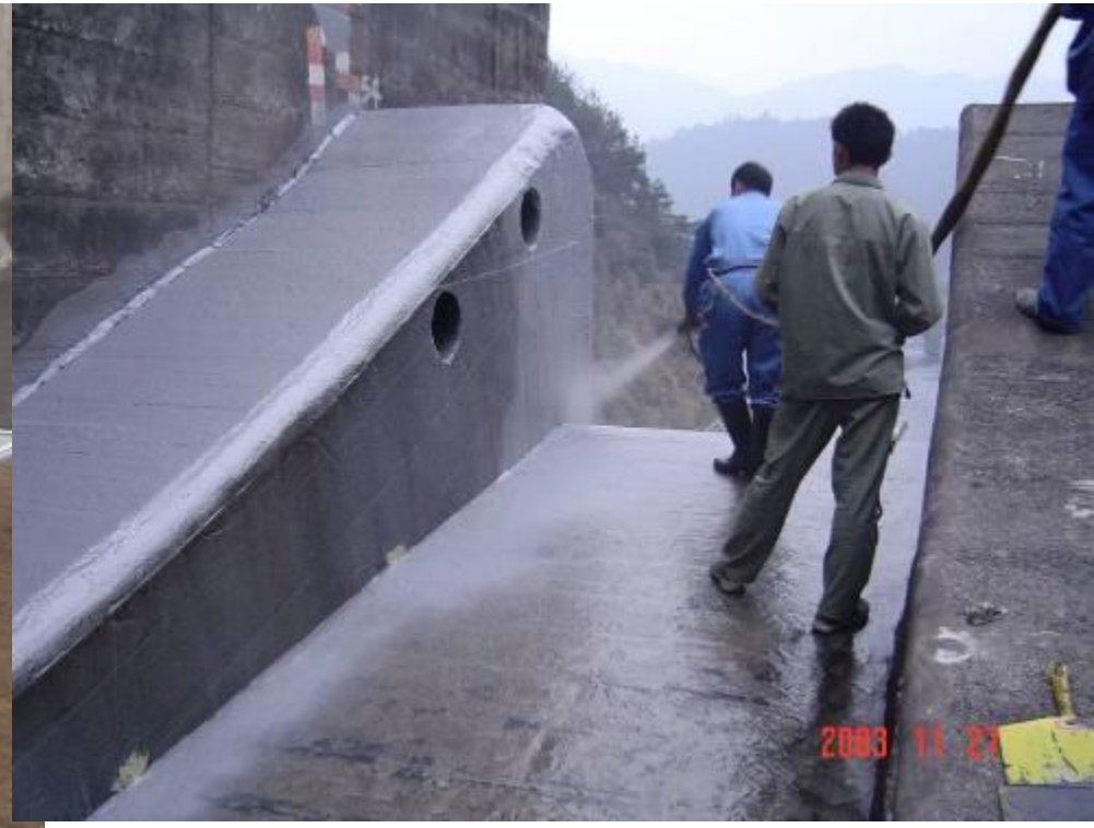
Anti-abrasion of flood flush in reservoir
